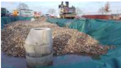
Fig. 3 Betonnen infiltratie put in systeem
